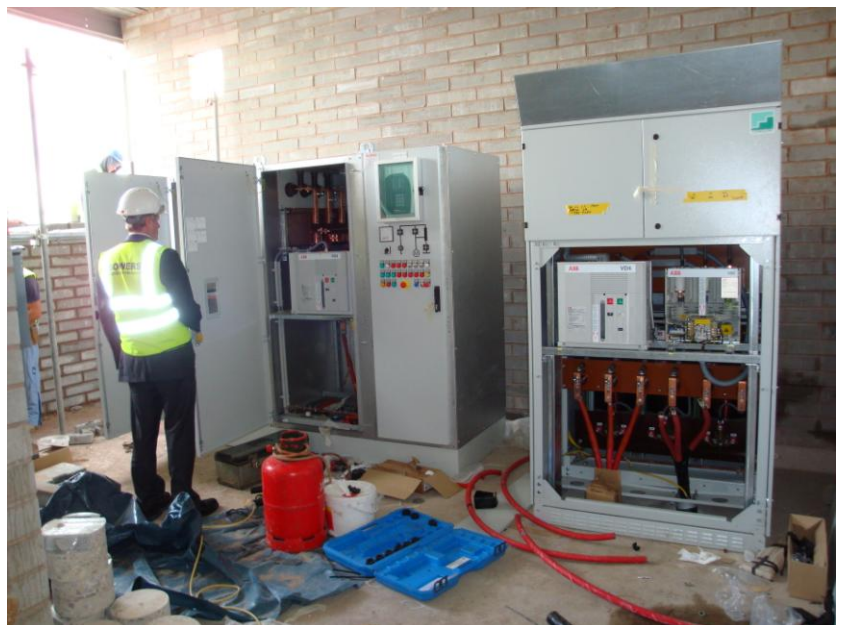
Motor control System being installed
