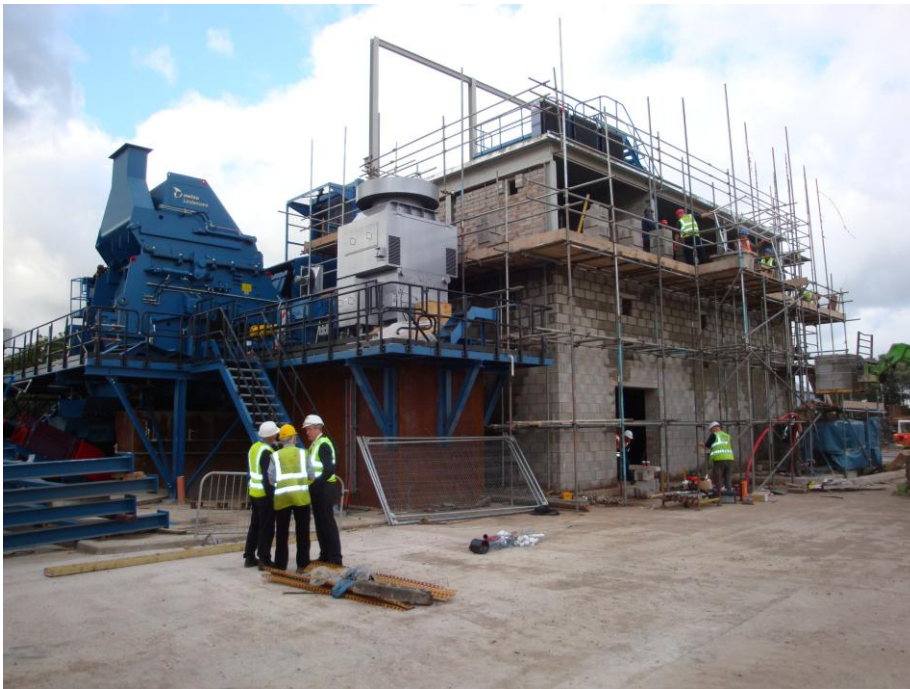
Picture of Main Crushing Plant During Manufacture with 3000HP Crusher Motor in the foreground
