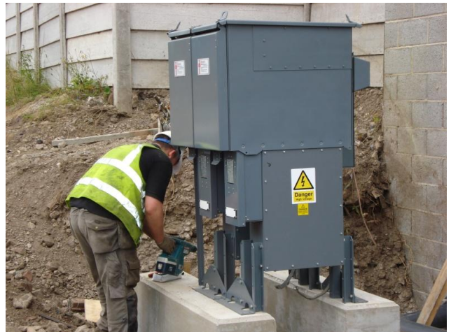
New 2 Panel Schneider 11kV Switchboard
