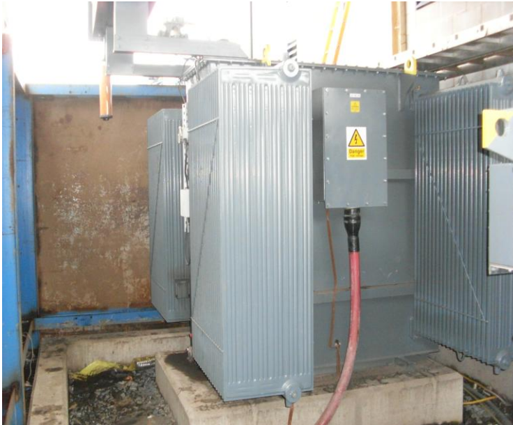
New Bowers 4500kVA 11kV to 433v Transformer being installed
