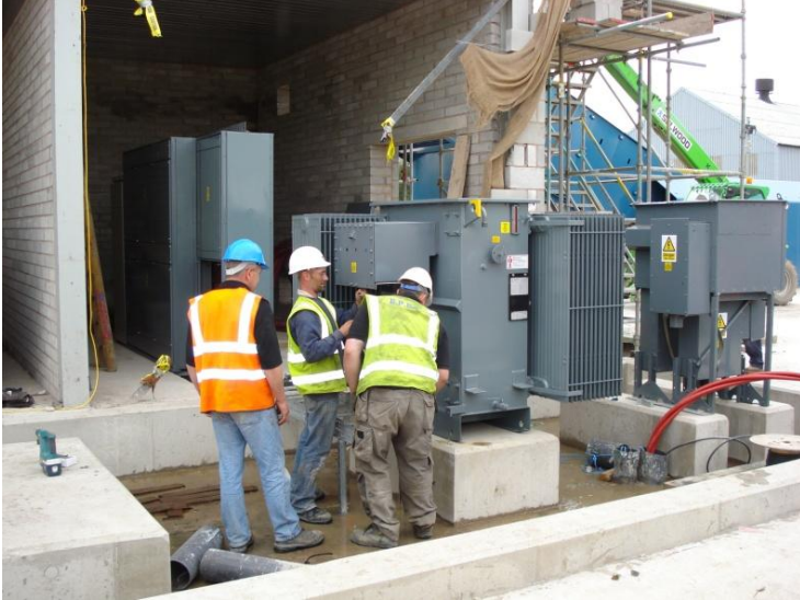
New Bowers 1250kVA Distribution Transformer
